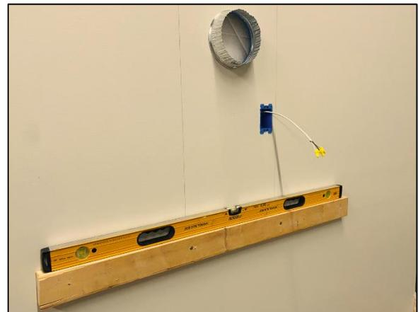
10. *With the weight of the hood, it is suggested to have two people lift hood into place on the cleat board.*
