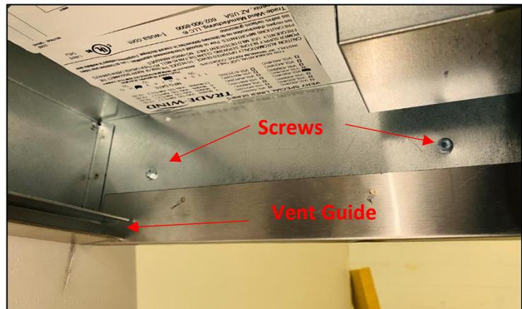
20. Install the air vents and center piece onto the blower unit.
