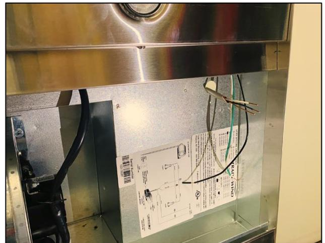
16. Using the appropriate electrical connectors, connect wires from blower unit to the home wire.
