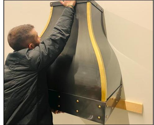
11. With hood in place double check hood is centered. Install at least four screws into the pre-drill holes.
