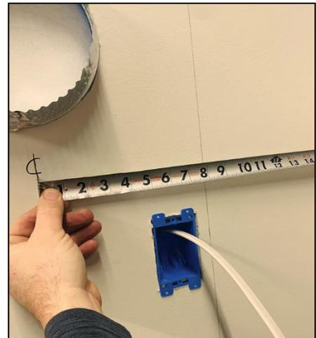
6. On the backside of the hood measure the width of the top and bottom of the hood and mark the center.
