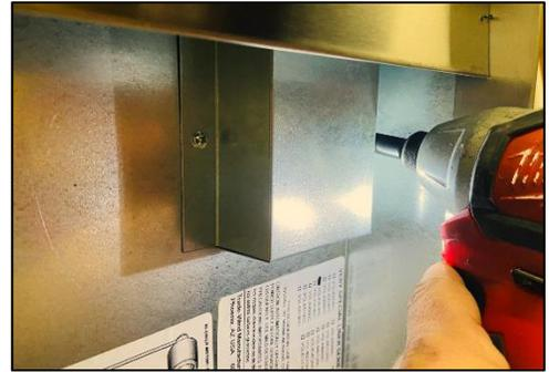
18. Connect the flex pipe to the plastic damper on the blower unit using ¼" self-tapping screws. (suggested 4 screws evenly placed around the duct). *Wrapping pipe to duct with foil-backing tape will also help ensure a tight seal.*
