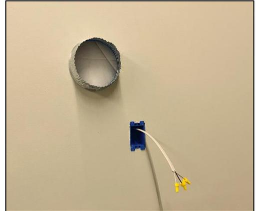
3. Using a stud finder locate studs to secure hood to. Once studs are located, you can use a level to mark the studs vertically to allow ease of locating studs to secure hood to the wall.
