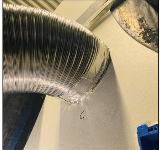
5. From the center of the duct, measure the distance to both studs located on the left and right side of the duct (*note these measurements as they will be needed when marking the studs location on the hood*)
