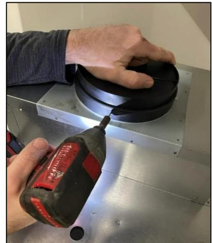
13. Place blower unit below the hood and temporarily support in place to allow ease of electrical and duct hook ups.
