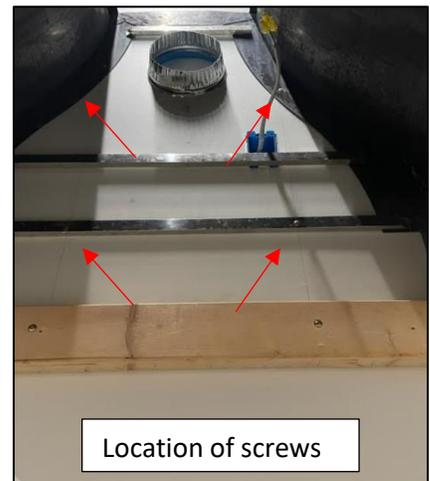
12. For the blower unit install, locate the plastic damper and install onto the vent of the unit using 1/4" self-tapping screws.
