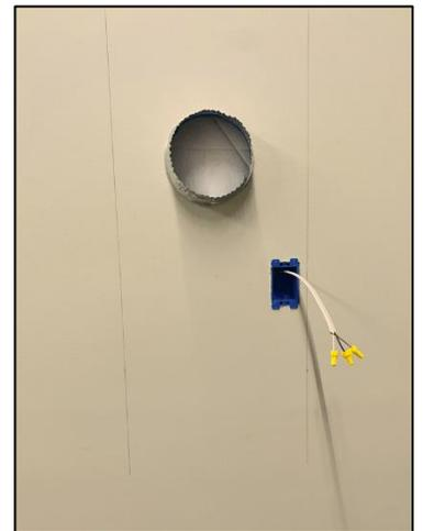
4. Install rigid flex piping onto the duct located on the wall and secure with 1/4" self tapping screws (suggested 4 screws evenly placed around the duct). *Wrapping pipe to duct with foil-backing tape will also help ensure a tight seal.*
